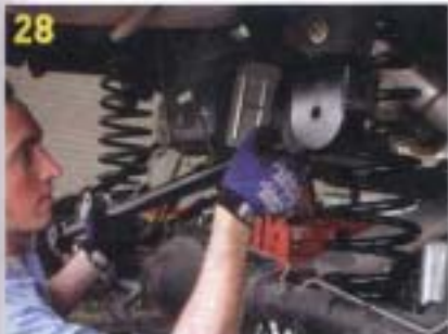
THE NEW ADJUSTABLE FORWARD BAR BOLTS IN ITS NEW LOCATION THANKS TO ANOTHER DROP DOWN BRACKET.
